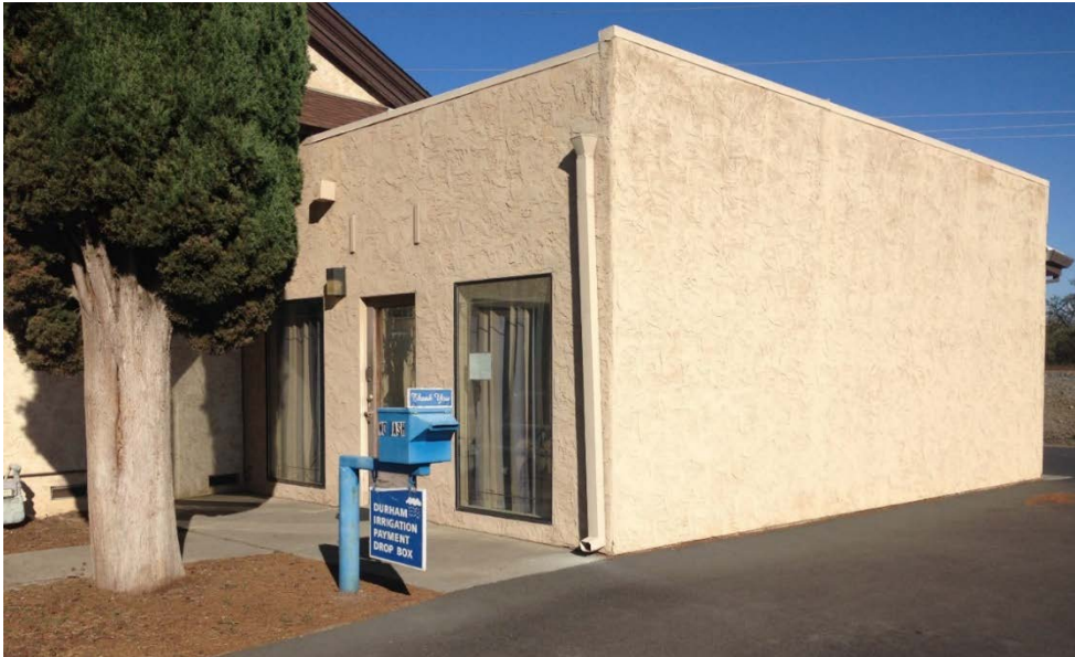
Figure 3 Durham Irrigation District Office
